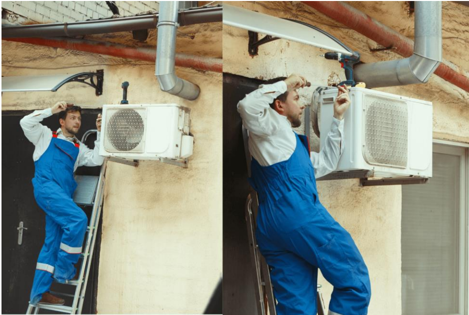
Figure 23 Maintenance of Air Conditioning [26]
